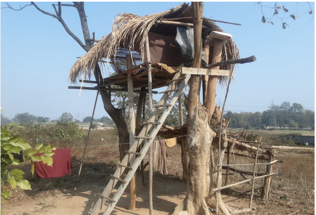
Figure 46: A locally made watch tower on a tree to guard and protect the crop from elephants
