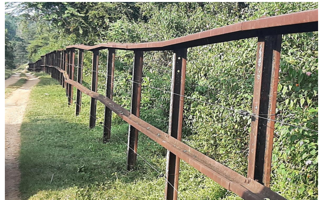
Figure 50: Picture of a rail barricade fence installed in Karnataka, India, Photo Credit: THG Pvt. Ltd.
