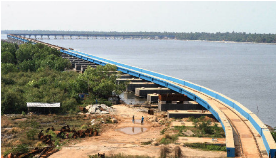
Figure 3: Construction of Railway Bridge along the Cochin backwater
