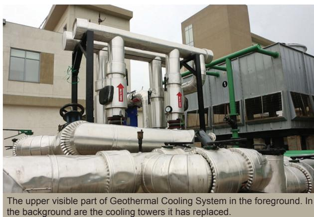
The upper visible part of Geothermal Cooling System in the foreground. In the background are the cooling towers it has replaced.
