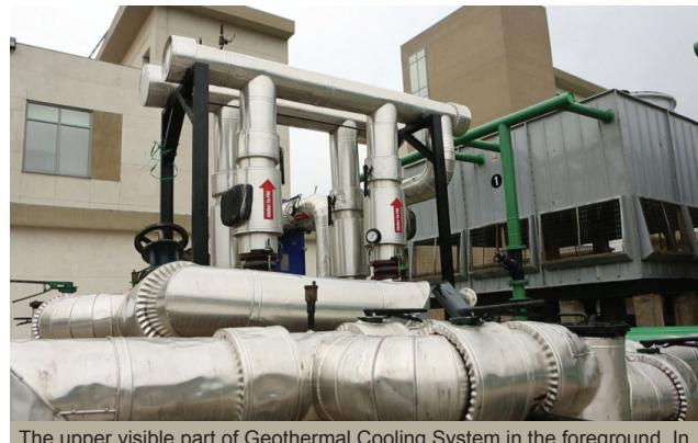
The upper visible part of Geothermal Cooling System in the foreground. In the background are the cooling towers it has replaced.
