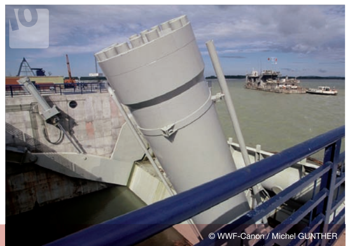
Lock gates at Gabčíkovo Dam on the Danube River, Slovakia.
